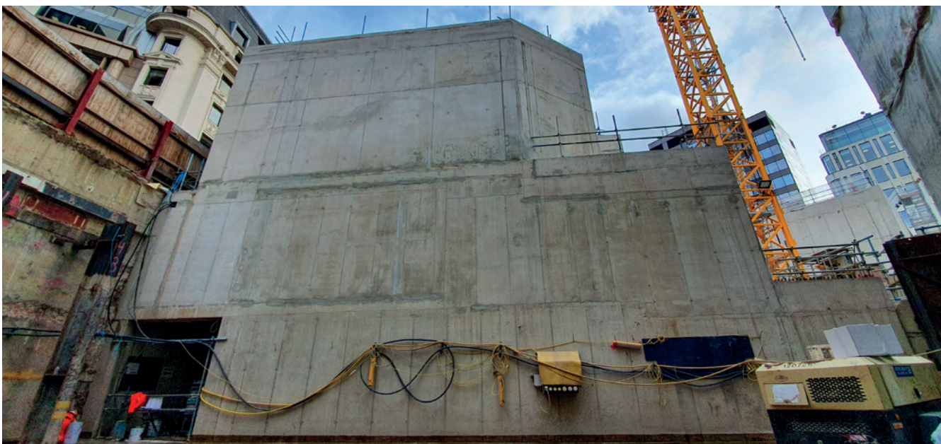
Bank Station Capacity Upgrade, London. Image courtesy of Sika.
